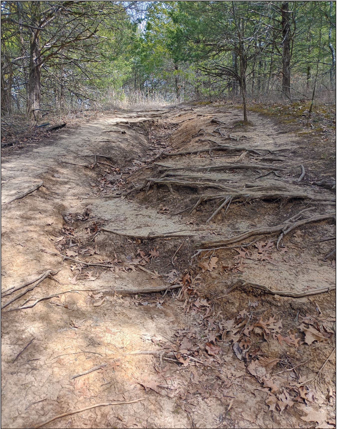
Figure 4. Adjacent to the GCRA is Rock Bridge Memorial SP where this often-traveled trail is showing significant signs of erosion from mountain bike use. This is an image of the Spring Brook Trail which is near Devil's Icebox Trail and can be difficult to traverse by average hikers.
